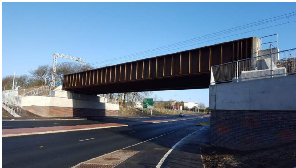
Fig 1. Rail Bridge founded on conventional pile groups.
